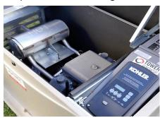
2. Locate the generator circuit breaker and the generator switch. The breaker is above the controller. The switch is on the controller and will have multiple settings OFF/AUTO/RUN.
