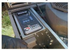
2. Locate the generator breaker and the generator switch. The switch is on the controller and will have multiple buttons OFF/AUTO/RUN. The breaker is located on the front of the controller cabinet.
