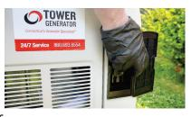
in the on position and close the lid. If the generator was not in an outage situation or running, you may turn the switch and the breaker on without a pause in between. This completes the process.
