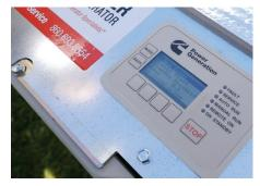
2. Locate the generator breaker and the generator switch. The switch is located on the controller and the breaker is located behind a black door on the right front of the unit.
